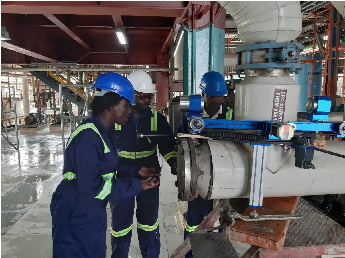
Team mounting CT gantry on sludge line
